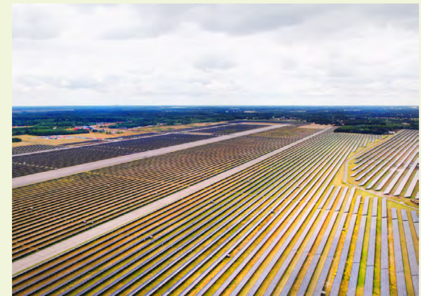
Vandel III, a utility scale solar photovoltaic park is located in the Municipality of Vejle in central Jutland, Denmark
